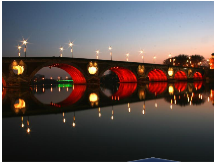
Pont-Neuf (Toulouse in France)
