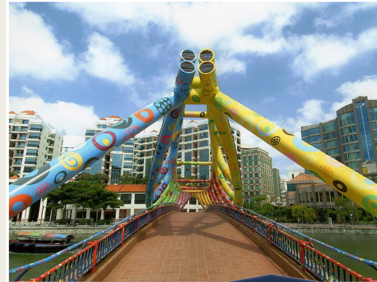
Alkaff Bridge, Singapore
